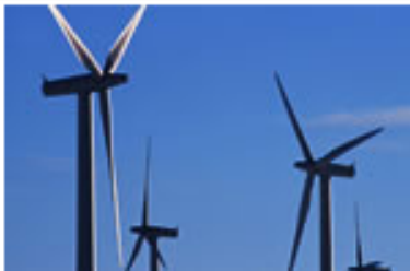
Innovative WIND TOWER Power Generation
